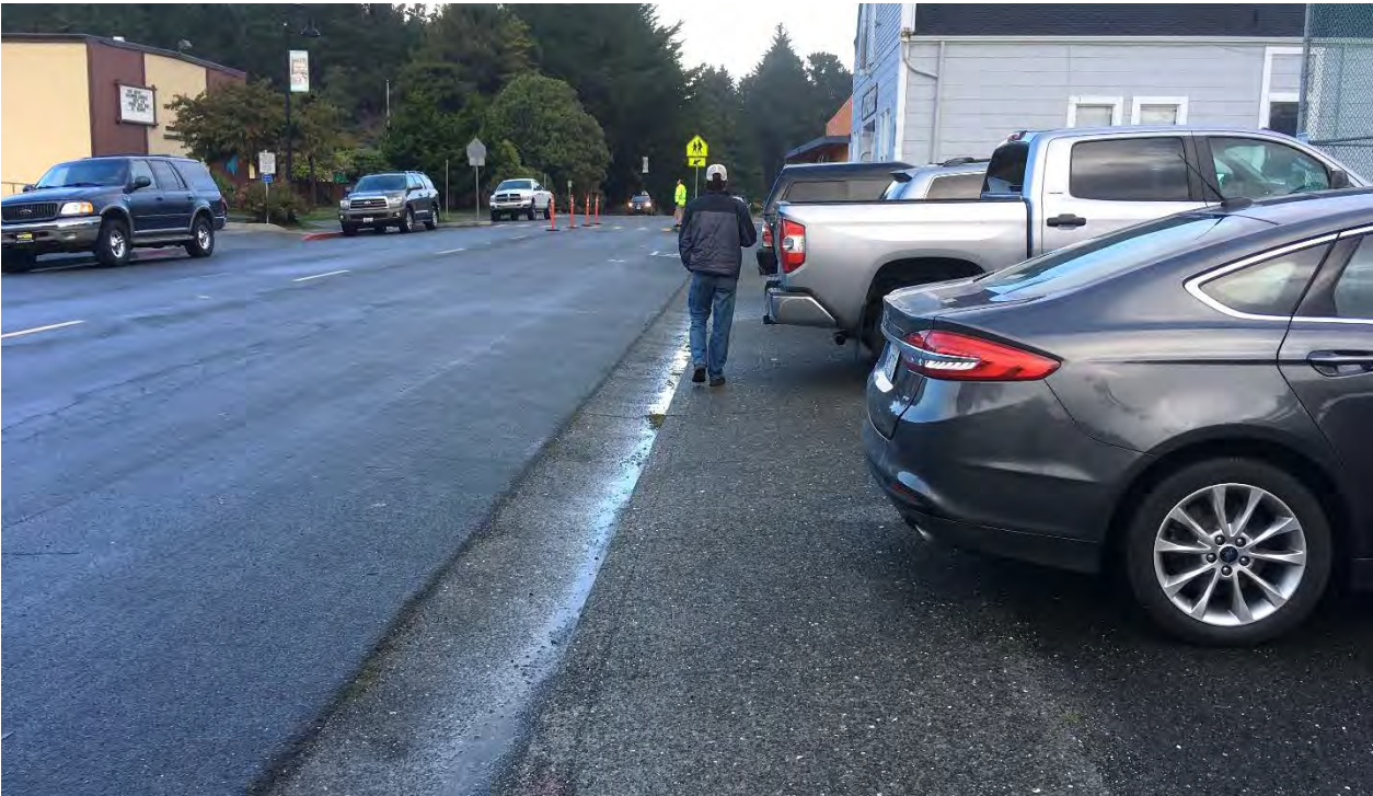
Sidewalk/driveway blocked by off-street parking (Trinidad Elementary School and Town Hall in background). Driveway is also non-accessible/non-compliant with cross-slopes greater than 4%.
