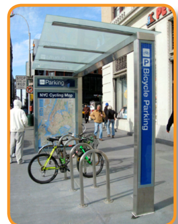
Figure 2-32: New York City project to install 37 new covered bicycle shelters around the city using standard bus shelter design (photo: AllWaysNYC.com)
