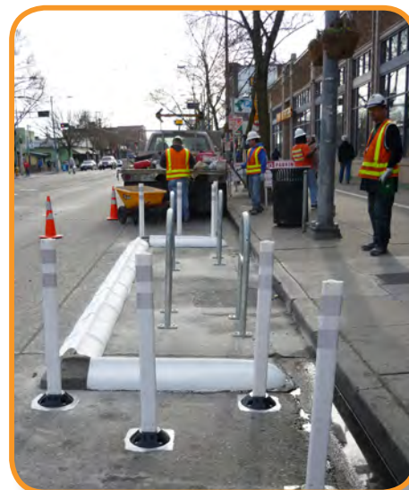
Figure 2-38: Concrete curbs are used to encourage entry from the sidewalk and protect bicycles (photo: City of Seattle, Wash.)
