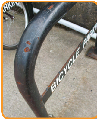
Figure 2-3: Powder coat (photos: Dero Bike Racks; Andrew J. Besold; figure: Dero Bike Racks)
