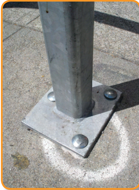
Figure 2-14: Flange concrete rack mounting (photo: Eric Anderson)
