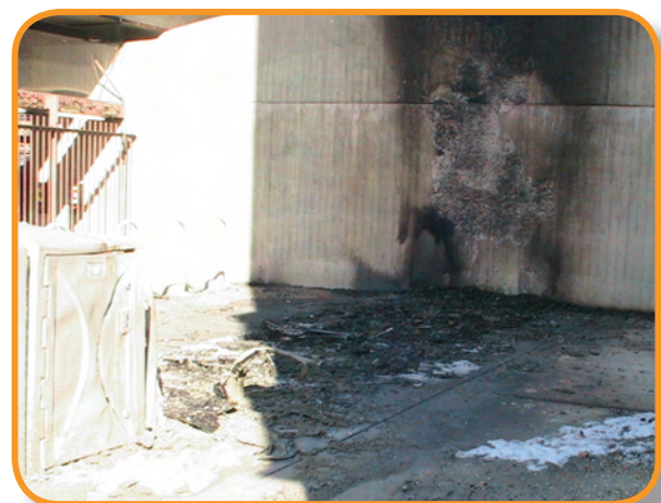
Figure 2-10: Molded polyvinyl or polyethylene lockers are susceptible to fire damage (photos: Laura Timothy, BART)
