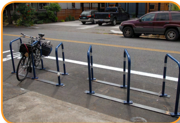
Figure 2-36: Inverted U racks are welded in clusters of three onto steel tracks in order to affix to an asphalt surface (photo: Jonathan Maus, BicyclePortland.org)
