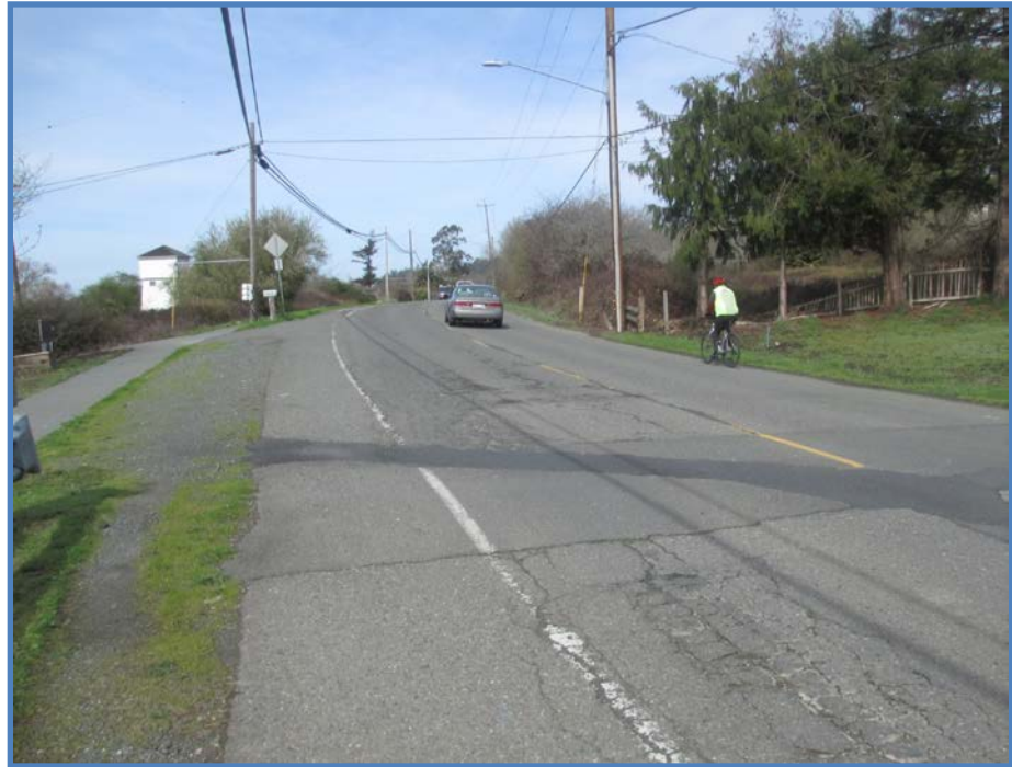
Figure 2.1 Image of the Old Arcata Road showing the road’s current condition and the separated path (SHN et al., 2017).
