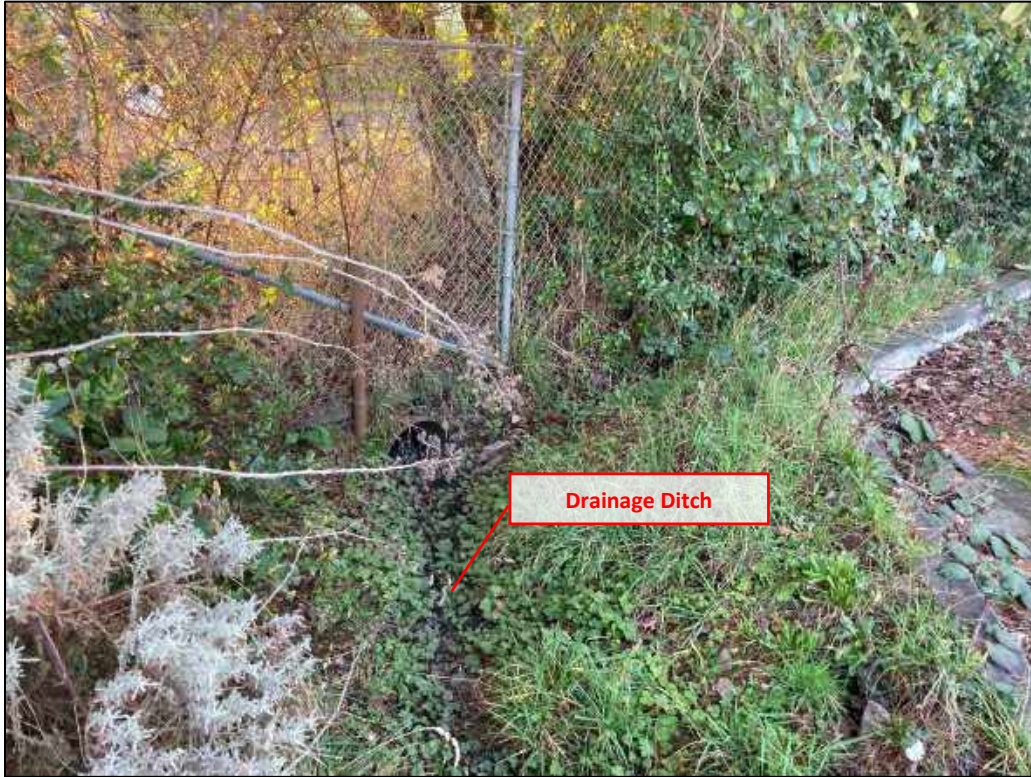
Photo 7: Drainage Ditch (Storm Drain Improvement #2)
