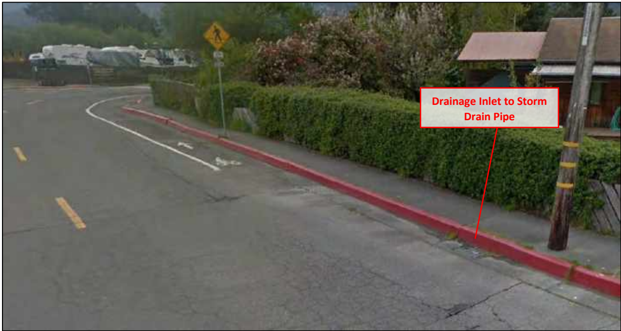
Photo 1. Drainage Inlet (Storm Drain Improvement #1)
