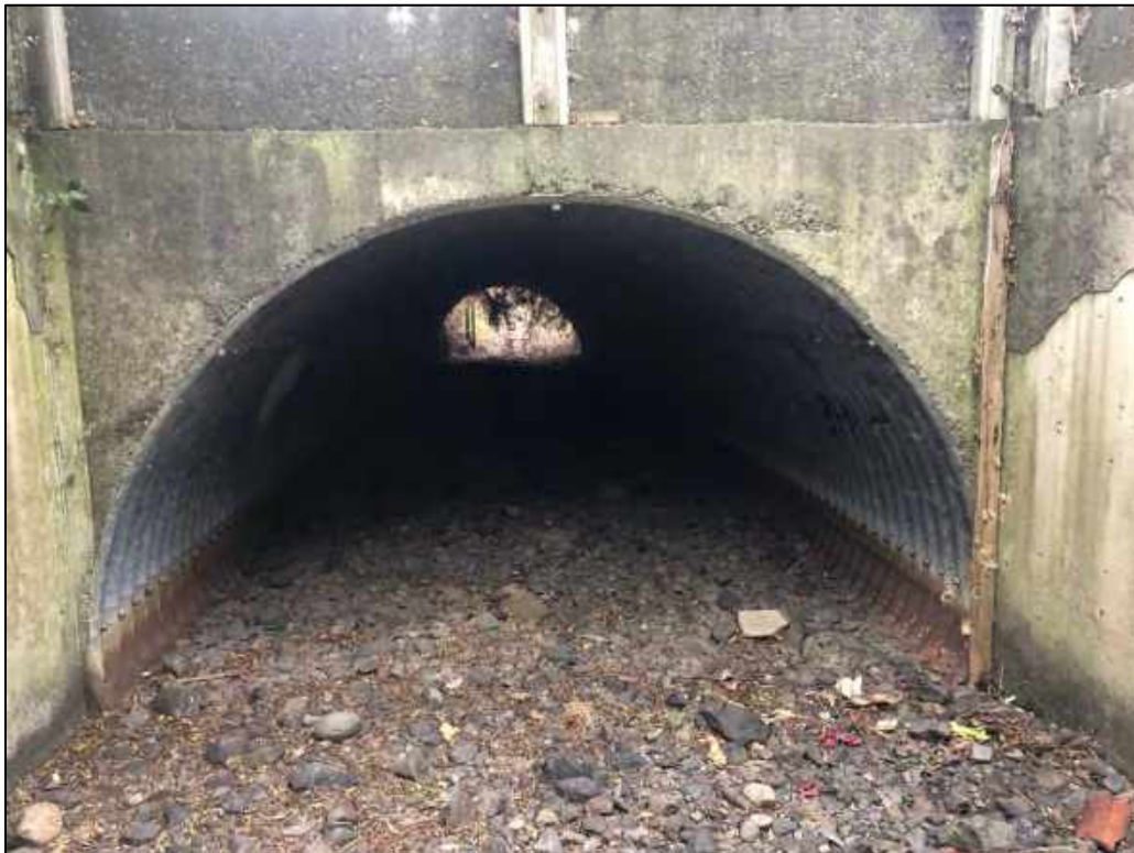
Photo 4. Inlet of CMP Arch Culvert (Storm Drain Improvement #1)
