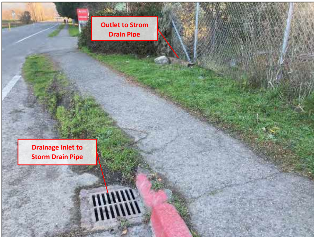
Photo 6: Drainage Inlet (Storm Drain Improvement #2)
