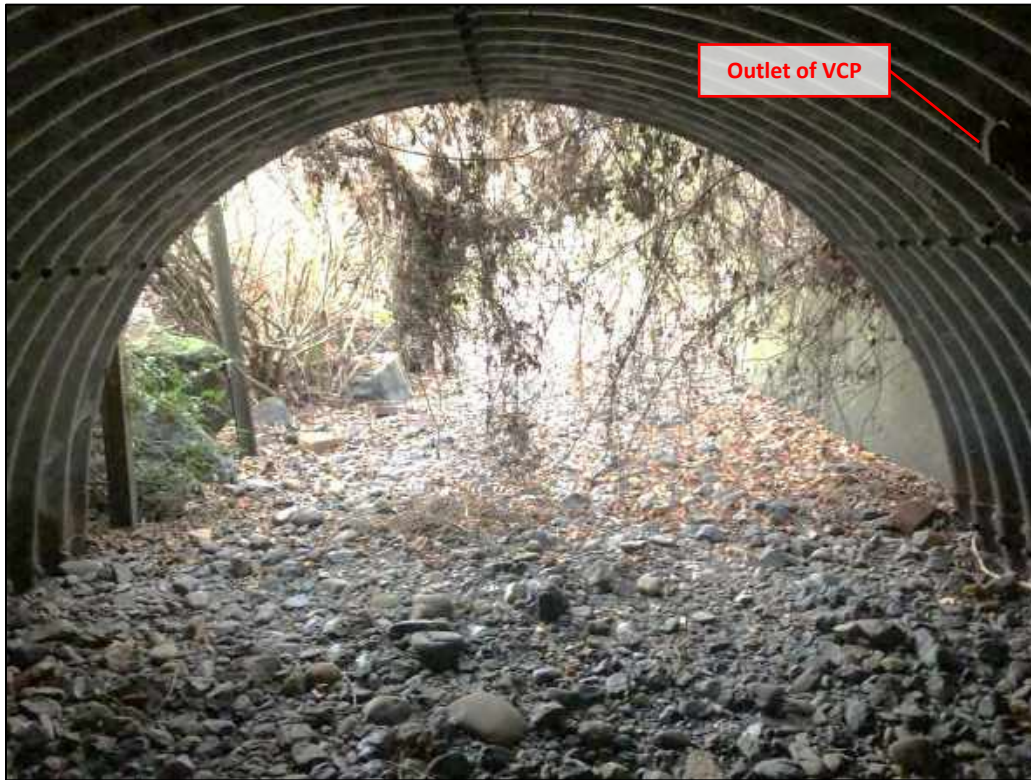
Photo 5. Outlet of CMP Arch Culvert (Storm Drain Improvement #1)
