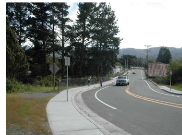
Sidewalks and bike lanes accommodate non-motorized travelers on Chartin Road.
