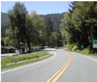
Highway 96 through Weitchpec has no pedestrian facilities despite frequent pedestrian activity.
