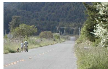
Pedestrians are forced to walk in the travel lanes on Hatchery Road.
