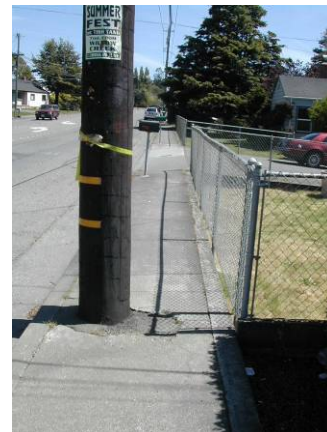
The photos above of various routes in Myrtle town display a variety of sidewalk obstructions, ranging from permanent impasses to temporary vegetation, all of which represent a significant obstacle to pedestrians with special needs.
