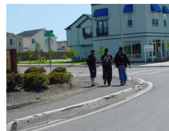
An asphalt “dike” provides some protection from vehicles.
