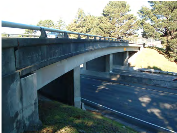
12 th Street Overcrossing - Looking East
