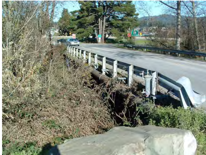
Strong's Creek Bridge on Riverwalk Drive – Looking East
