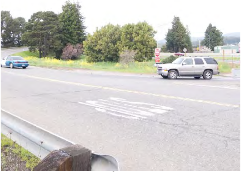
Southbound Hwy 101 exit ramp at 12 th Street, looking NE
